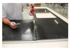
4. Place the tops together and remove the silicone residue with washing-up liquid.
