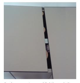
Apply connectors and lightly push the worktop into position.
