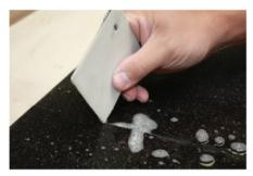
5. If there is a joint cut into the butt of the top, then hold the spatula with the point downwards (as shown in the picture) in order to remove the surplus silicone. Then clean the worktop according to the care instructions.
