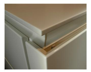
Fix recess grip with external corners (Silicon).
