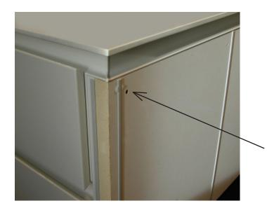
Screw end panel support frame to the connecting carcase.
