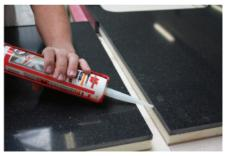
2. Apply silicone to the joint on edges to be joined.
