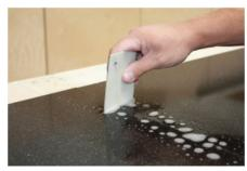
If the butt is without a joint, then just run the straight edge of the scraper over the worktop to remove the rest of the silicone.
