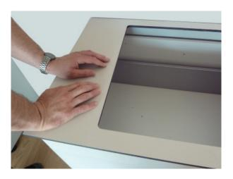
Press down and remove surplus adhesive. Clean joint surface.
